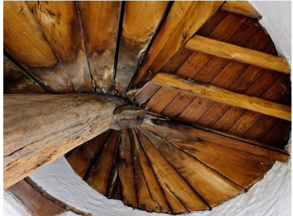
Spiral staircase at Eastbury manor House
